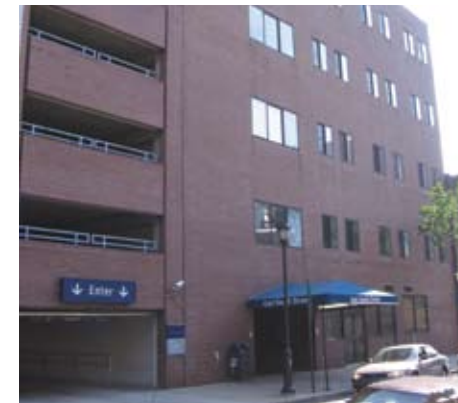
1740 South Street. The building's entrance, lobby and other public spaces were redesigned. Building mechanicals and all finishes were upgraded.
